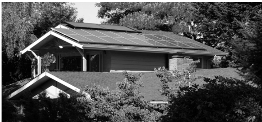
Solar water heating and photovoltaics on a Portland residence.
