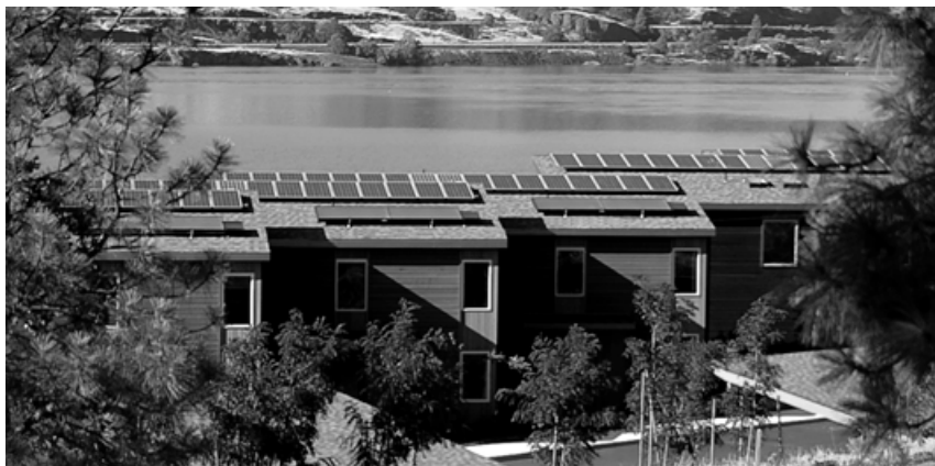
Solar water heating and photovoltaics on a condominium project near Hood River, Oregon provide 1/3 of all energy needed.
