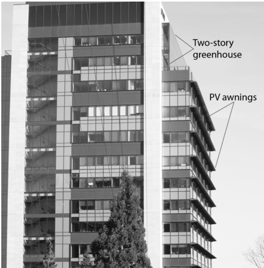
Photovoltaic modules double as awnings in the summer. The two-story greenhouse heats domestic hot water.
